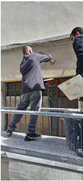
Applied by hand, like traditional plaster.
