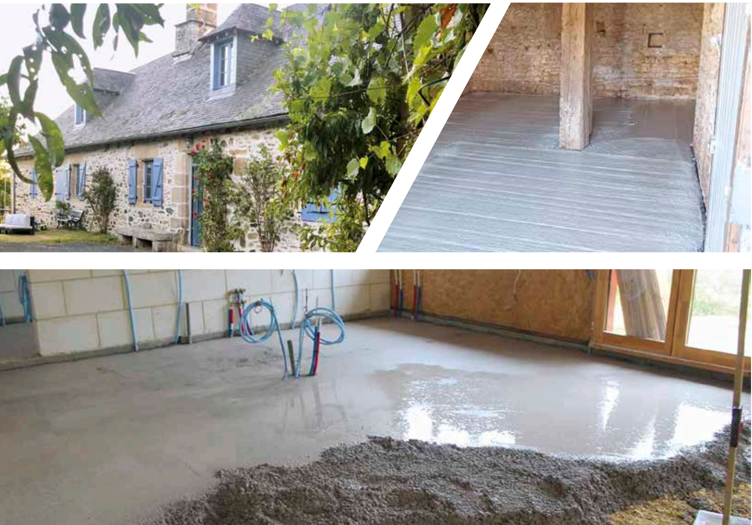
Limecrete paving with natural pozzolana aggregates, on tamped hardcore limestone. Private house (France).
