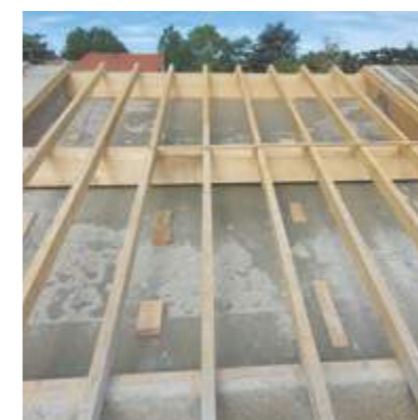
View of the roof formwork before filling.
