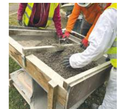
Hempcrete roof insulation.
