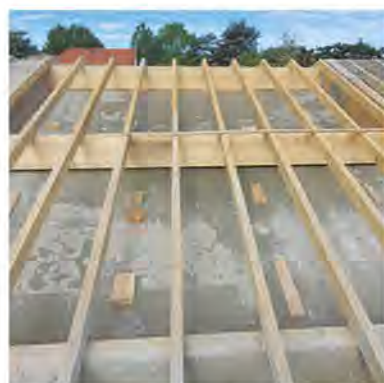
View of the roof formwork before filling.
