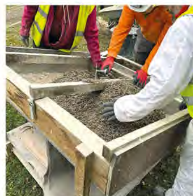
Hempcrete roof insulation.
